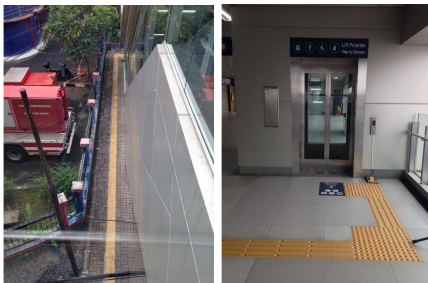
Figure 2& 3. Guiding tiles at Jakarta MRT Lebak Bulus Station
